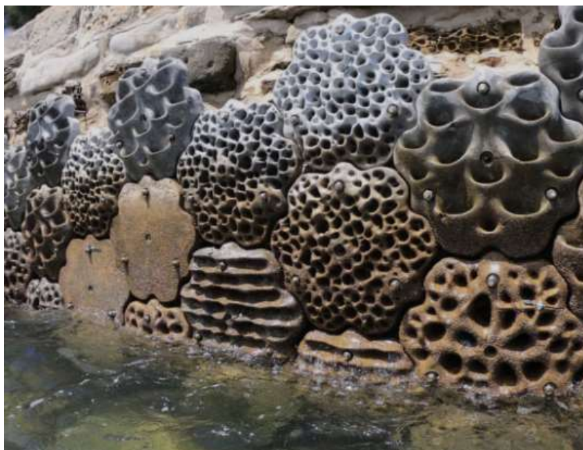
Figure 4-92: Example of aquatic plates to be installed on bridge abutments
