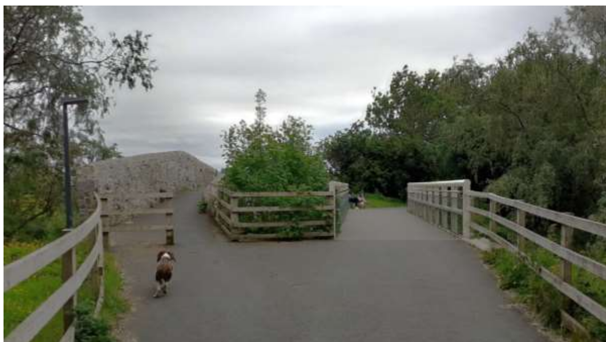
Figure 4-1: Existing Bridge at River Groody
