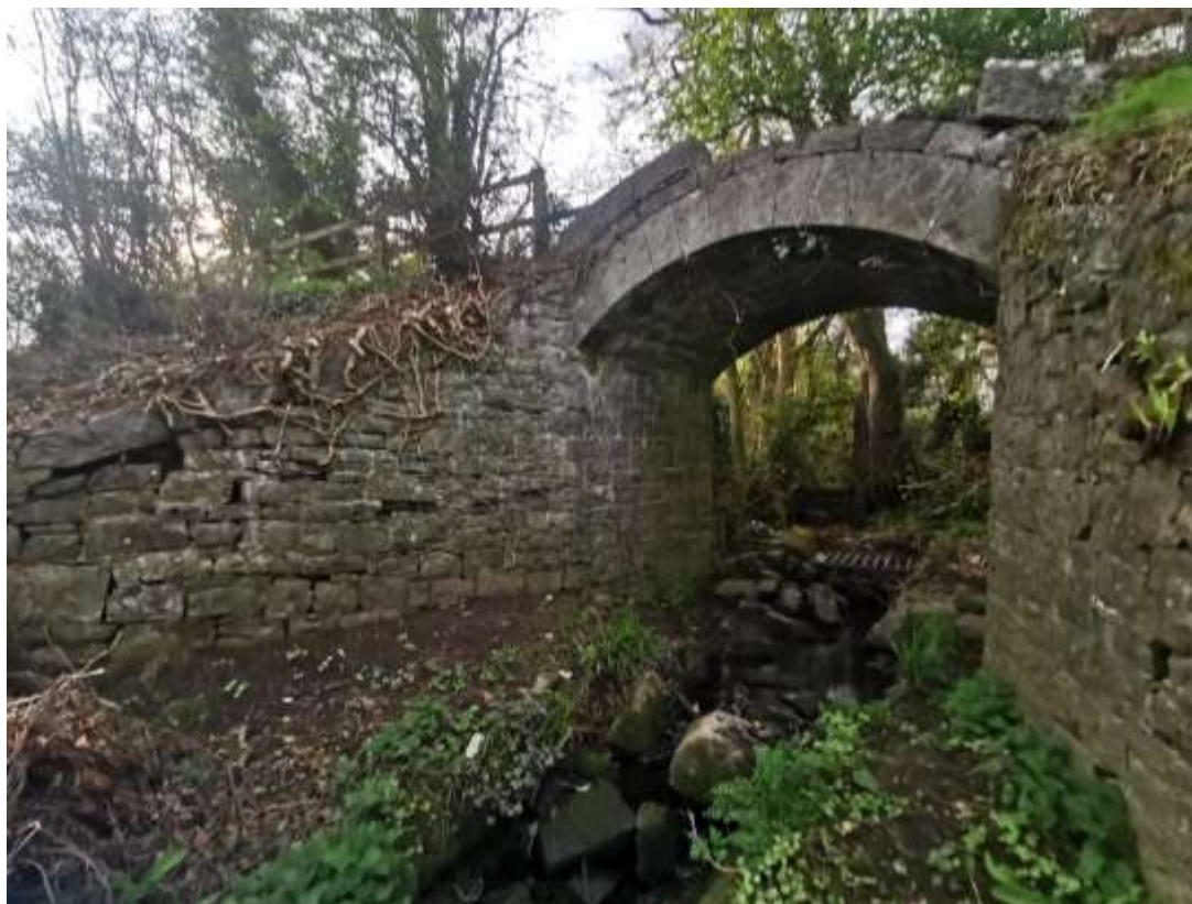
Figure 4-17: View of Bridge 2 from bank of drain
