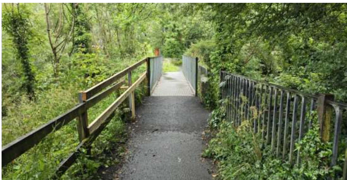
Figure 4-20: Existing temporary bridge across the Plassey mill race where it rejoins the River Shannon
