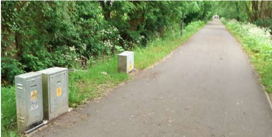
Figure 4-4: Existing path to be resurfaced
