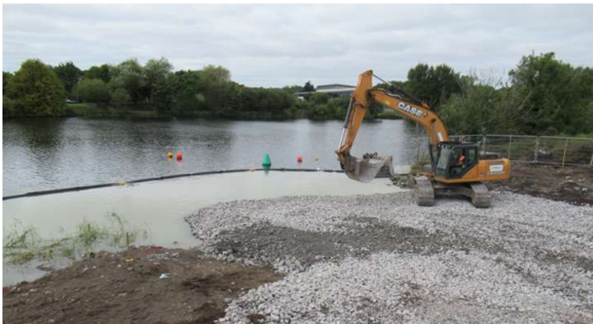
Figure 4-86: Silt curtain retaining contaminated water during advanced works for sheet piling
