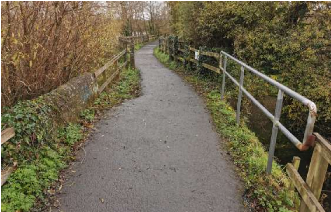
Figure 4-11: Existing bridge over land drain (Bridge 1)
