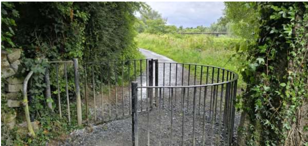
Figure 4-33: Existing kissing gate at the Garrison Wall to be retained on the gravel path that runs in front of the Fisherman cottages
