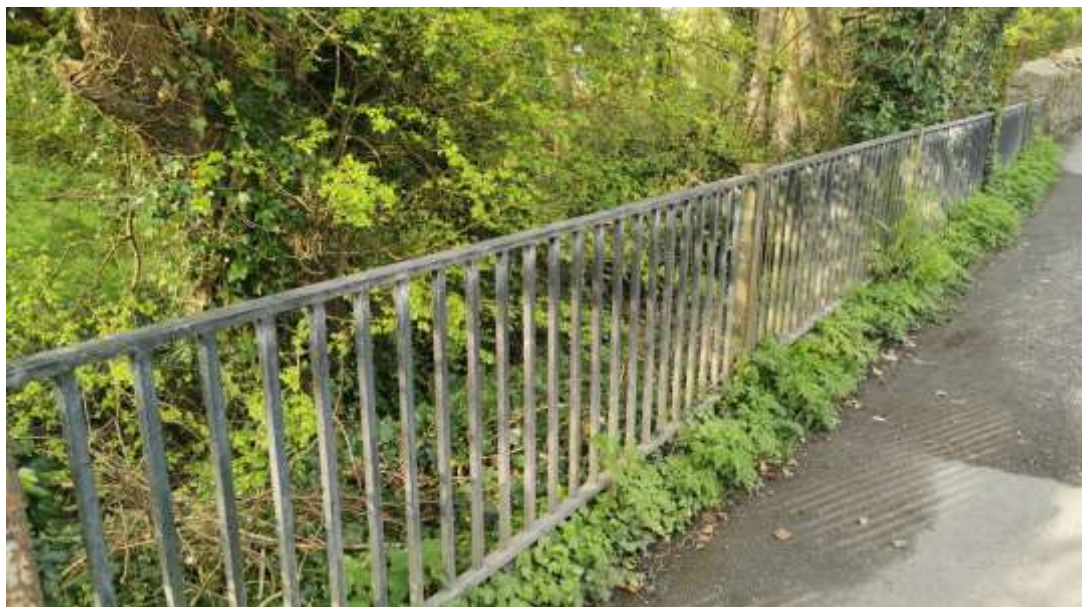
Figure 4-19: : Existing railing between Bridge 2 and Bridge 3
