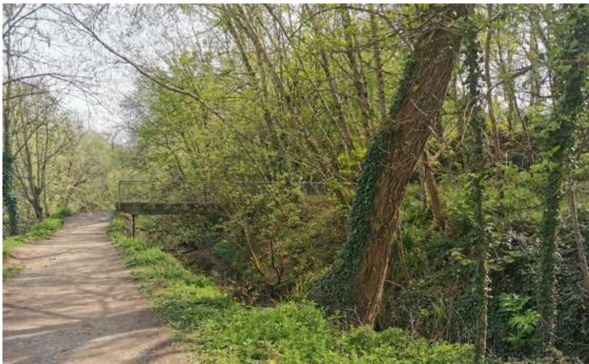
Figure 4-48: Existing concrete bridge at mouth of Plassey mill race (to be retained)
