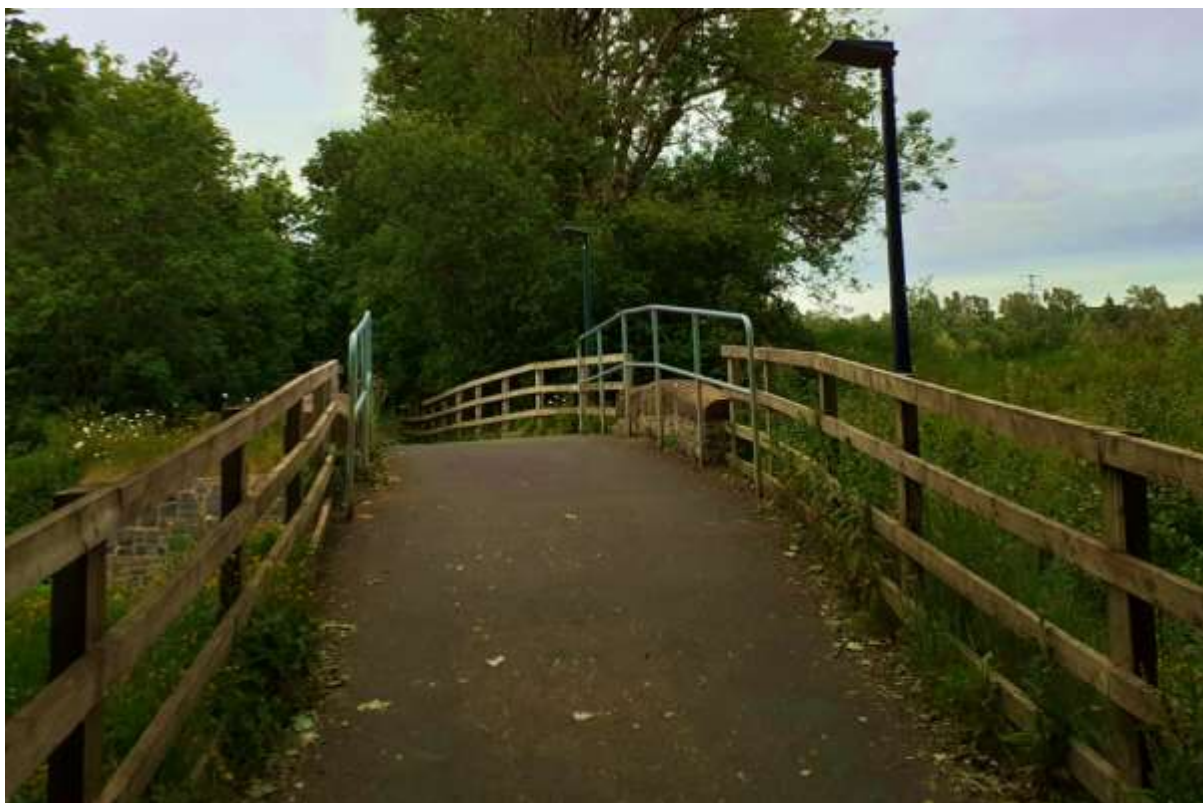
Figure 4-78: Existing bridge at CH400
