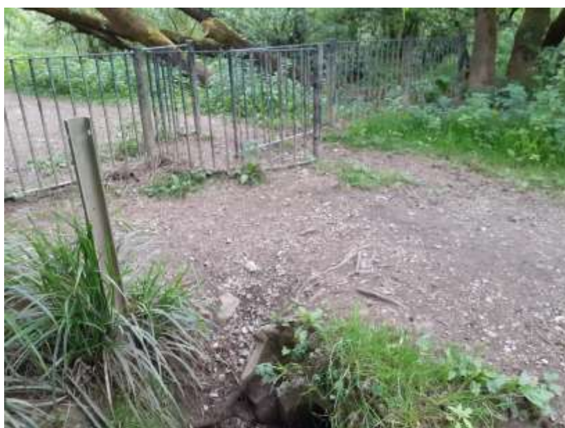
Figure 4-54: Existing gate and culvert at the land boundary between UL and the IDA
