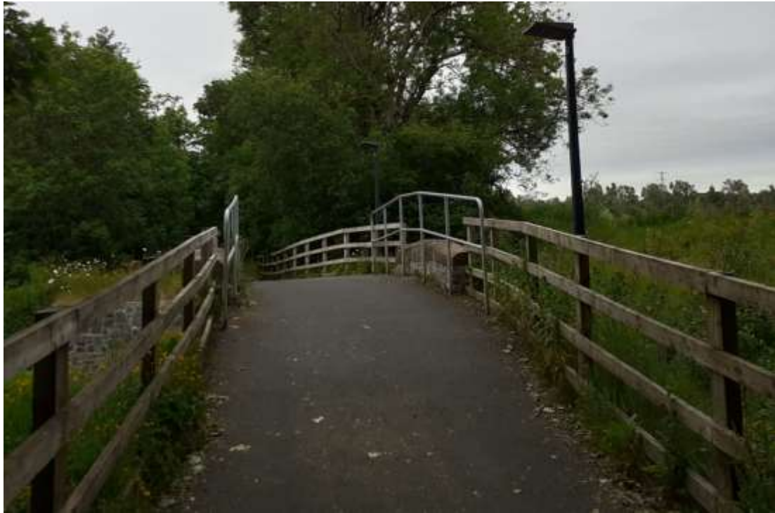
Figure 4-3: Existing bridge at CH400
