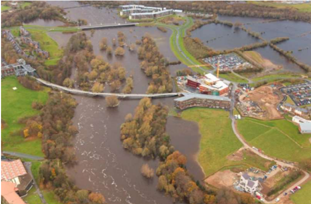
Figure 4-137: November 2009 River Shannon Flood Event at UL campus in Co. Limerick on left hand side, with UL campus in Co. Clare on right hand side of figure, OPW database ( www.floodinfo.ie )
